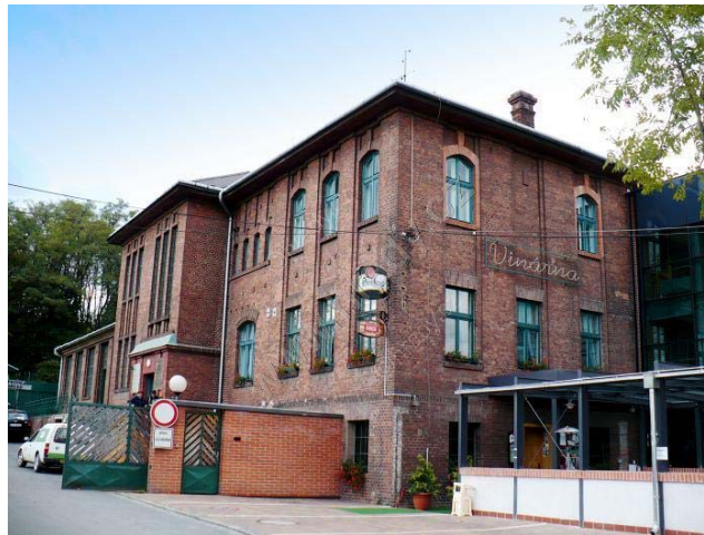
Former mine Jan Maria in Ostrava (Czech Republic) – rebuilt for new pub and hotel
