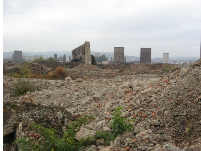
Former iron works in Hunedoara (Romania) – demolitions as start of redevelopment?
