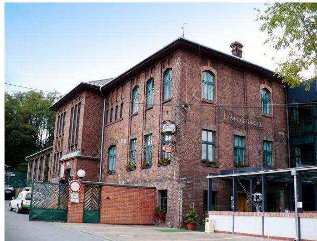
Former mine Jan Maria in Ostrava (Czech Republic) – rebuilt for new pub and hotel
