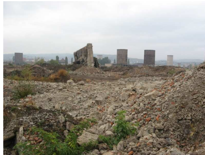
Former iron works in Huneduora (Romania) – demolitions as start of redevelopment?
